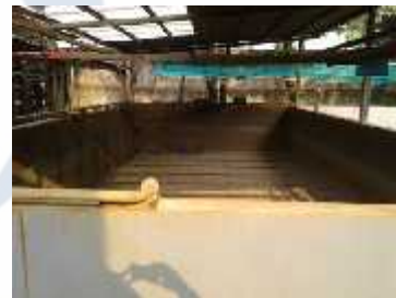
CLEAN WATER POND
